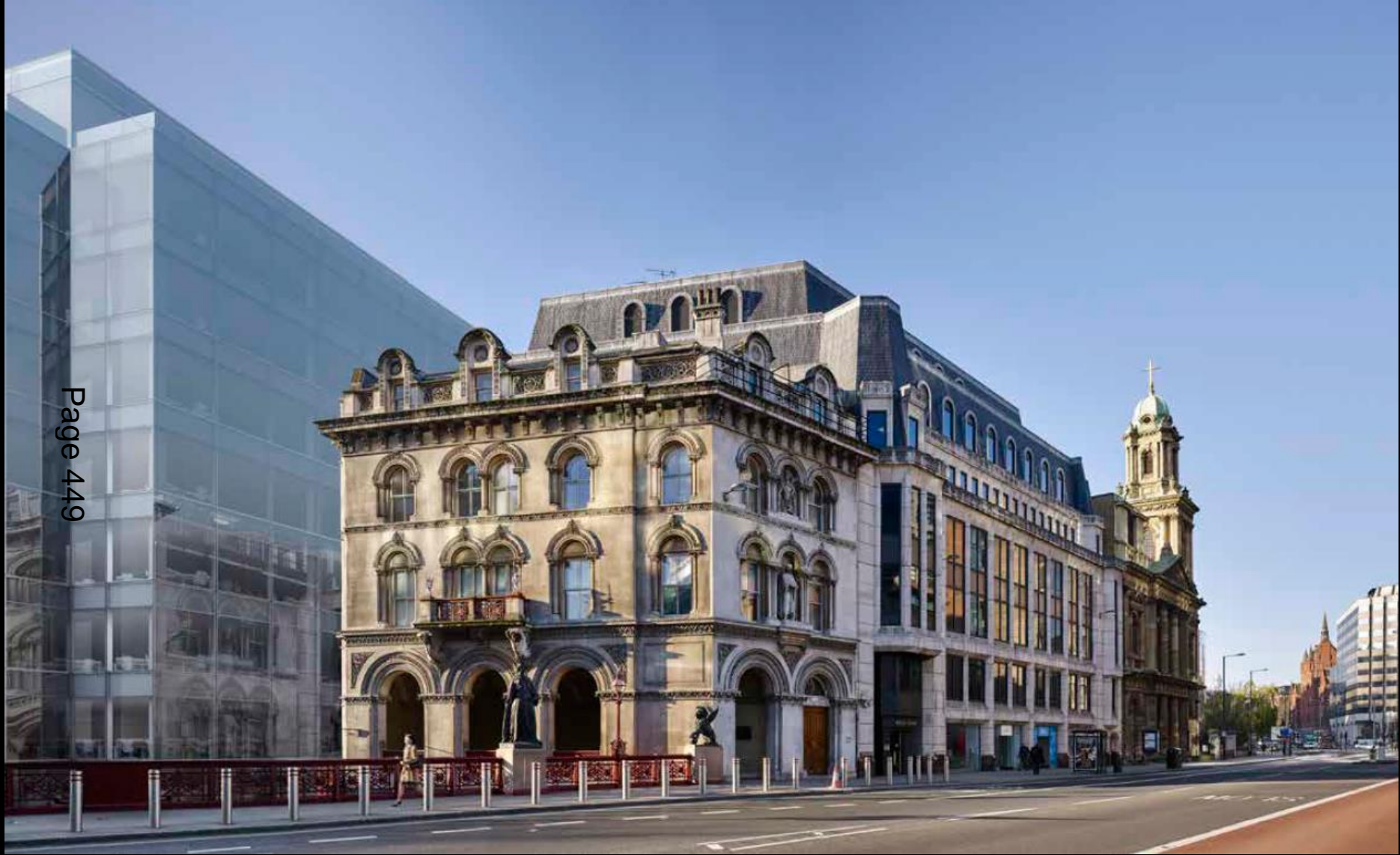
Existing north-east view
